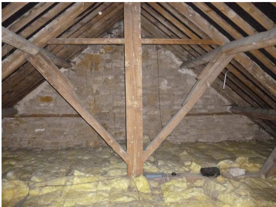
King-post roof structure
